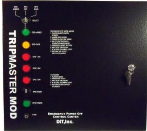
The TripMaster MOD (Modular) Emergency Power Off Control Center (EPOCC) is designed to handle heavy switching loads with field selectable versatility to provide the best EPO solution for any facility. The EPOCC simplifies designing EPO control systems by providing individual relay outputs for as few as 4 outputs to as many as 20 isolated high current relay outputs different systems in the data center.
